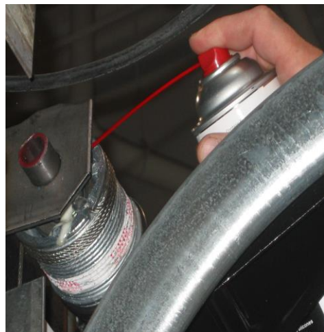
CABLE DRUM BEARING
