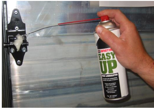
END HINGE PIN & ROLLER SHAFT
