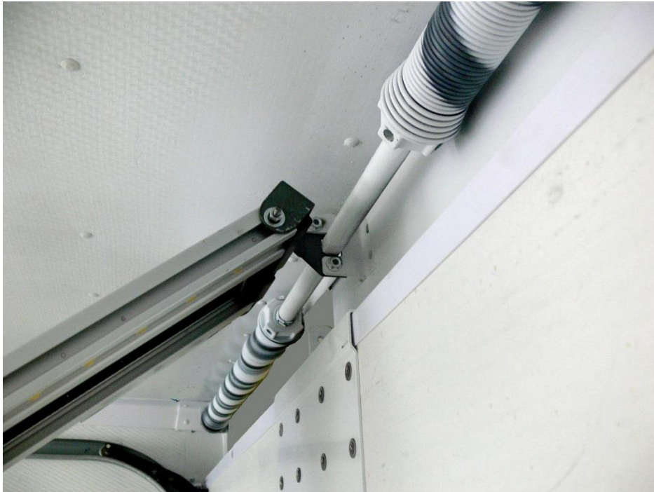
Connecting the track to the header
